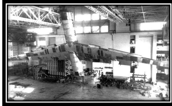
A B-36 airframe undergoing structural stability tests.
