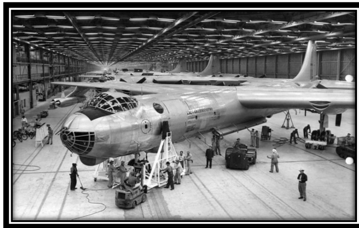
RB-36s in production. Note the heavily-framed "greenhouse" bubble canopy over the cockpit area, used for all production B-36 airframes.
