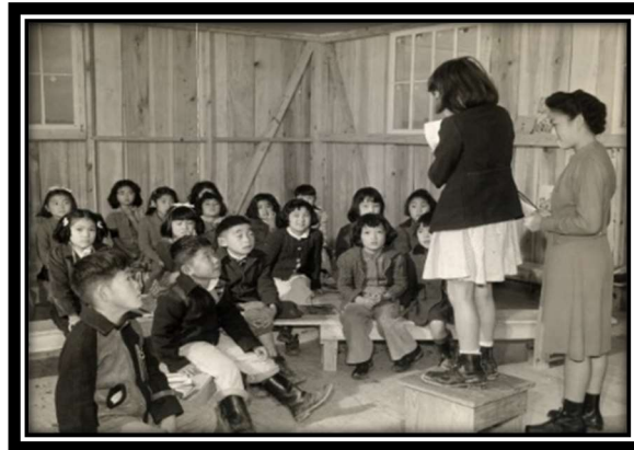
One of the Classrooms
