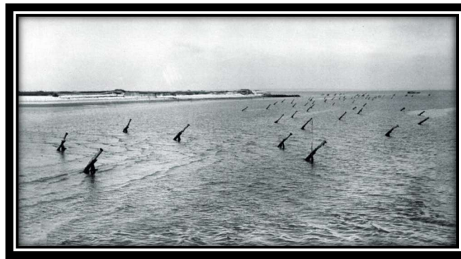
This photo taken at low tide off the coast of Normandy shows devices known as "Rommelspargel" (Rommel's asparagus): German teller mines attached to posts. These were designed to be concealed below high tide and destroy landing craft. (National Archives)
